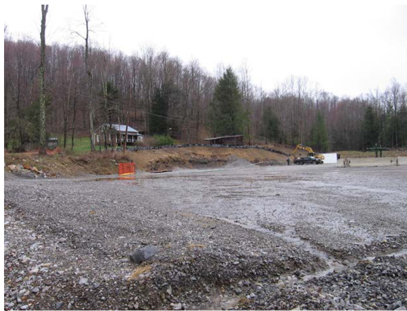
Finished wellsite with its neighbor.
